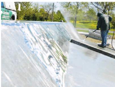
PHOTO: QMI AGENCY Goodbye Graffiti technician Ramrah Singh uses pressurized water and cleaning solution to remove graffiti at the skateboard park at Coxwell and Lakeshore.
